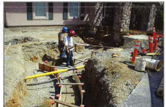
Workers construct rebar footing for the gift shop expansion (an addition of 1,712 square feet) at Seven Feathers Hotel & Casino Resort.
