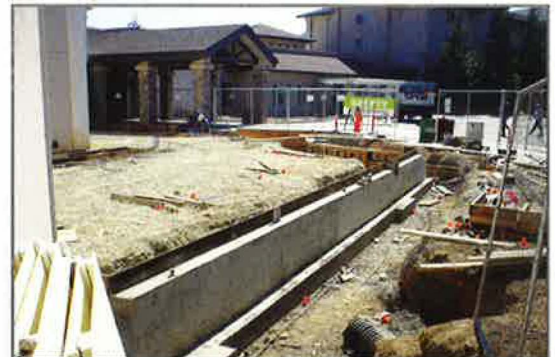
Completed stem walls for the non-smoking casino floor (an addition of 3,517 square feet) at Seven Feathers Hotel & Casino Resort.
