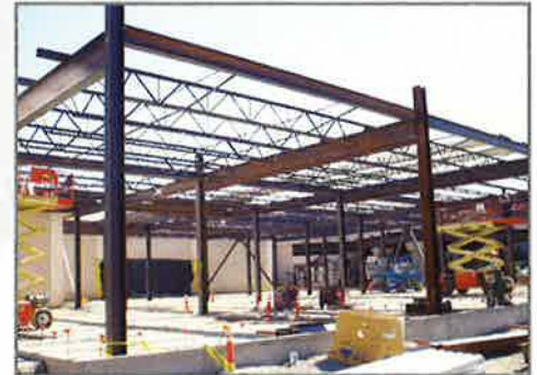
Steel and joist erection completed in early September as part of the expansion project at Seven Feathers Hotel & Casino Resort.
