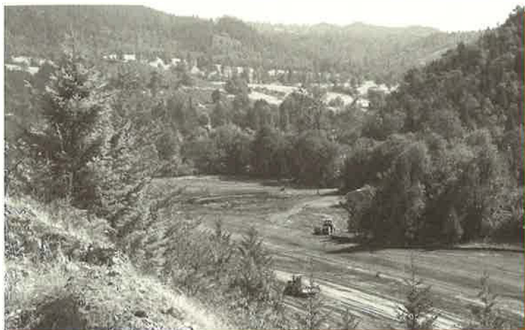
Erosion control is part of every day's activity. Silt fences are in place. Hay bales have been put down. Over 75 acres of land will be hydro mulched.
