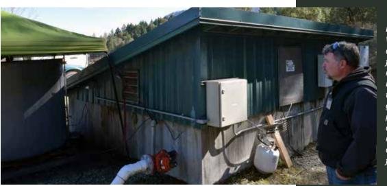
Left: UIUC Plant Operator Paul Wolford monitors the hastily assembled yet efficient mechanism for applying the PAC to the reservoir water. The longer the PAC has exposure to the water, the more it is able to reduce the geosmin levels in the water--a process that Wolford is improving all the time. Eventually, this mechanism will be replaced with a dedicated facility for treating water for geosmin in the future
